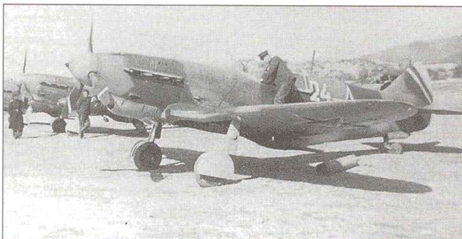
LaGG-3 'White 24' (a 66th Series machine) belongs to 9.IAP, VVS, ChF (Black Sea Fleet), who operated around Novorossiysk during the spring of 1944. The 66th Series was the last production version of the type, and it introduced considerable aerodynamic improvements over earlier versions. Further identifying features common to this version were four exhaust stubs and a small antenna mast. A 9.IAP LaGG-3 could usually be distinguished by its yellow-tipped tail fin and white striped propeller blades, as perfectly illustrated by this aircraft
